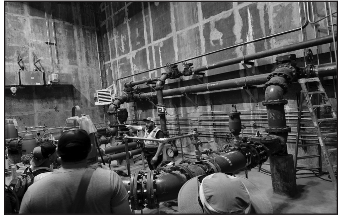
Figure 15. Pumping station for CSO 26 (combined sewer overflow tank 26), which gradually pumps the stored sewer-stormwater to the sewage treatment plant after the storm event passes.
